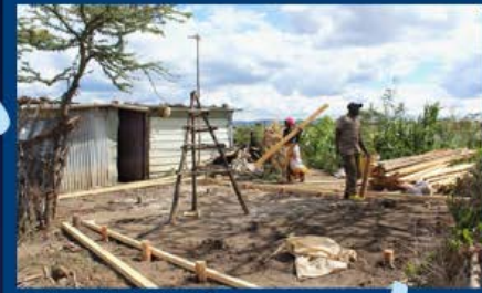
Laying the foundation.
