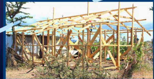
Building the frame of the house.
