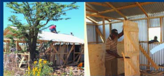
Left: Installing a leak-free roof; Right: Interior walls go up and a door is constructed.
