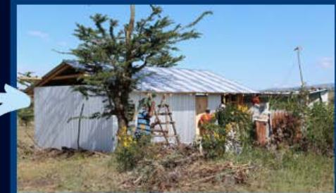
Siding and finishing touches!
