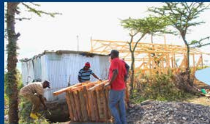
Installing the new pit latrine.
